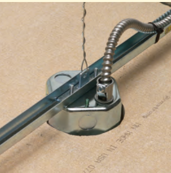
4 Cable pulled through cable connector (not supplied).
