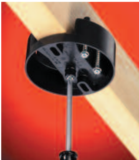
2 Tighten center screw to secure box to joist.
