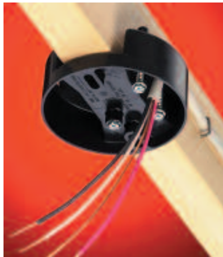
3 Pull NM cable through connector.
