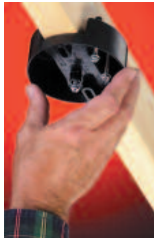
1 Press box onto joist.
