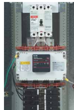
The SPD Series is also available as an integrated unit interfaced via a circuit breaker resident in the electrical assembly. This installation keeps connected lead lengths short while providing a means of disconnecting power to the unit quickly and easily.
