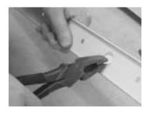
Step 3 Mount the 24R Plugmold base to the wall using No. 8 flat head screws every 32" max.
