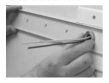
**Step 4** Cap wires at the end of the harness on both sides using wire nuts.
