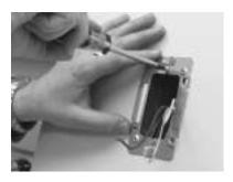
**Step 3** Cap wire at the end of the harness on the non-feed side using wire nuts.
