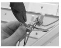
**Step 2** Feed cable through connector and attach the base to the 2451 or 1/2" trade size feed connector.
