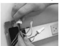
Step 2 Connect 24R Plugmold base to box or entrance end. Mount the 24R Plugmold base to the wall using No. 8 flat head screws.
