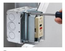
03 Re-tighten... Adjustment screws.
