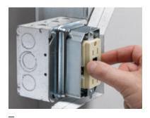
02 Adjust... Inner ring to be flush with wall surface.
