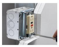
01 Loosen... The 2 adjustment screws located in opposing corners of the mud ring.
