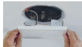
Friction clips for recessed housings
