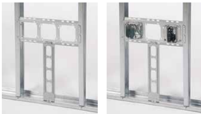
BBFS-18 Installed (can be used with BB7 or BB8 brackets)
