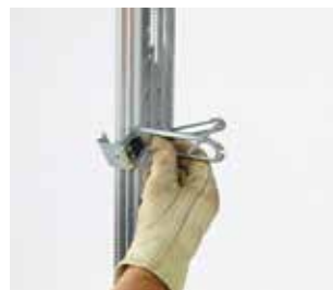
Push support onto stud
