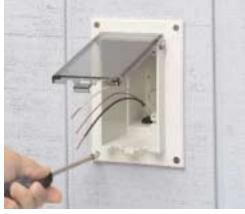
Attach IN BOX to substrate with tainless steel screws (provided).
