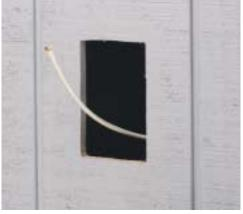
Note: Turn off power at the main panel box. Cut hole in substrate. Pull wiring.
