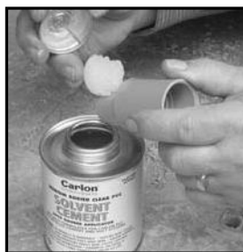
Apply a uniform coat of cement.
