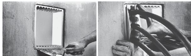
**1. Cast, grout or weld the one-piece mounting frame into masonry or steel surface.**
