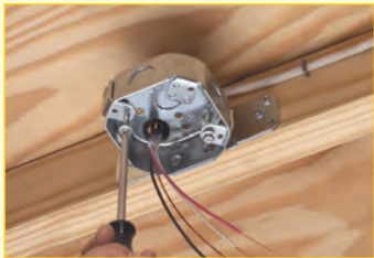
4 Install fan mounting bracket.
