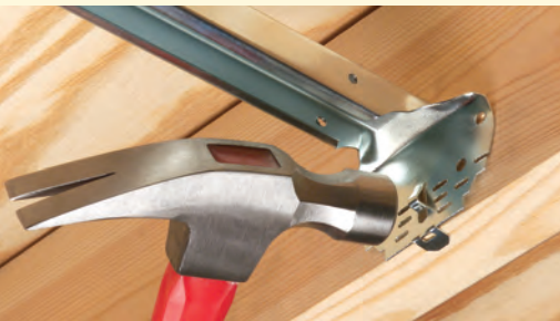
1 "Tooth" holds bracket temporarily in place.
