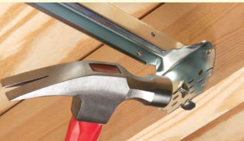
1 "Tooth" holds bracket temporarily in place.
