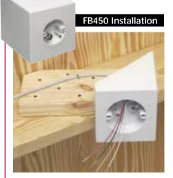
Cut a 2x8 approx. 18" long. Install FB450 on 2x8 allowing it to extend 8-10" past the box. Keep bottom of box level, short side of box touching angled rafter. Nail or screw assembly
