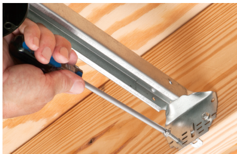
Bracket mounts securely to joists.
