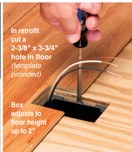
3 Adjust box height and install bracket
