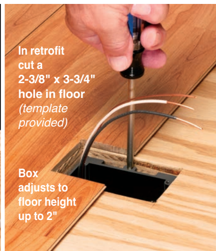
3 Adjust box height and install bracket
