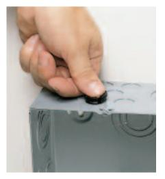
1 Push the NM cable connector into the knockout with light finger pressure.
