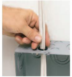
**2** Install one or two cables, fast! Push the NM cable (or cables) into the connector to the desired length.
