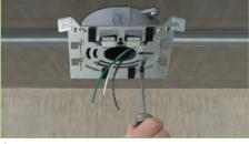
Step 1 Install quick mount bracket to wet location junction box.
