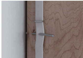
Inadvertent nails can puncture wire behind wall
