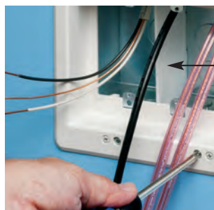
Mounting wings hold 2- and 3-gang boxes securely in wall.
