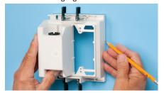
Use enclosure (without trim plate) as a template for opening. Cut hole.
