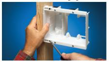
Attach box to stud using #6 screws. Use tabs on box for proper positioning of box depth.
