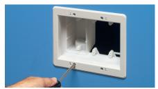
4 OPTION for new work: Tighten mounting wing screws to pull the box securely against the wall.
