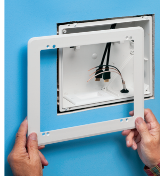
Attach trim plate with screws provided.
