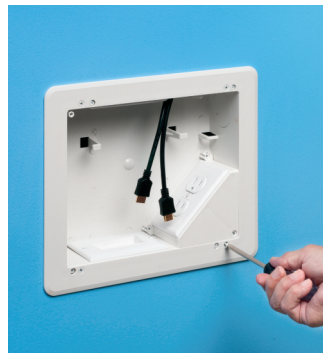
Pull cable. Tighten mounting wing screws to pull box securely against wall.
